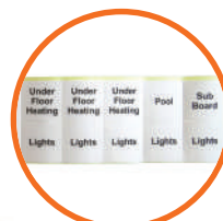
Label Circuits Clearly and Neatly for Easy Identification
